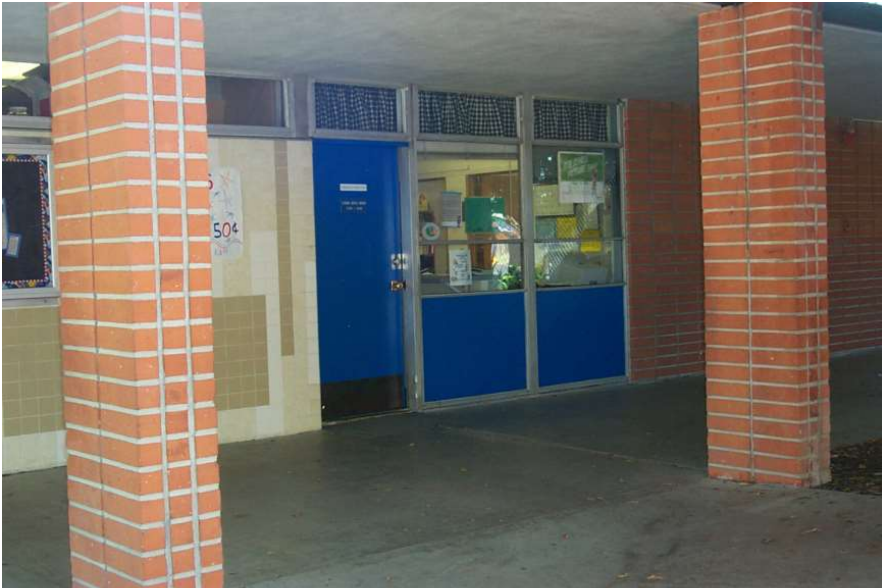
Disabled Building Access (ADA) – Beswick Elementary School
