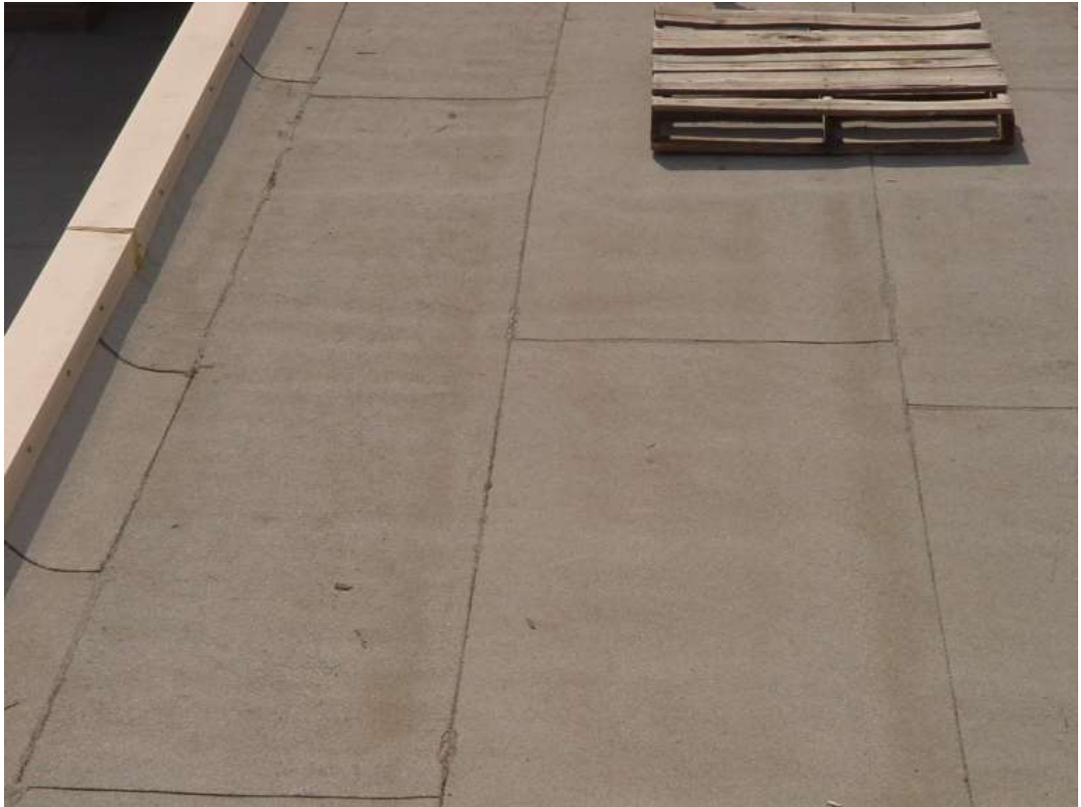
New Roofing – Myford Elementary School
