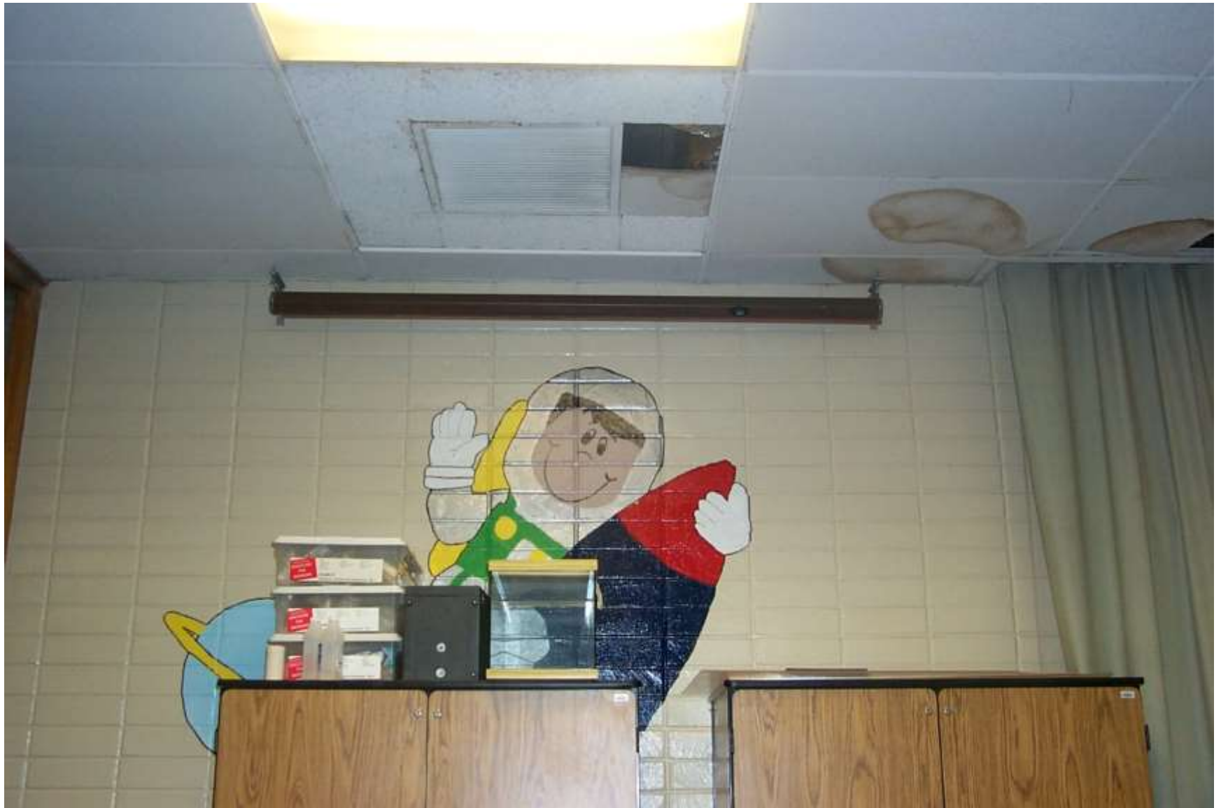
Building Integrity, Ceiling Repairs – Beswick Elementary School
