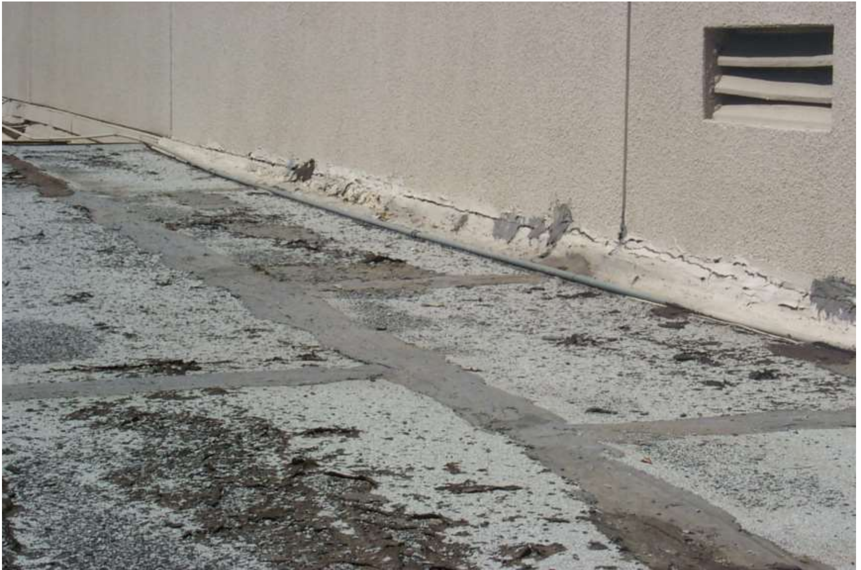
Building Integrity, Roof Replacement – Tustin High School
